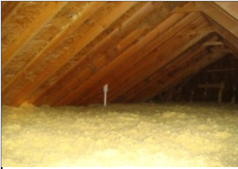
View of the attic.
