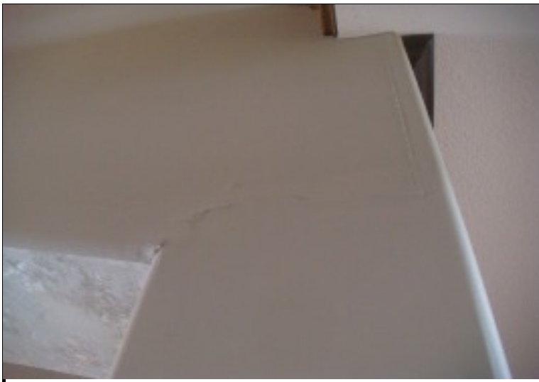
Repair cracked drywall surface at: Column at the main entry area.
